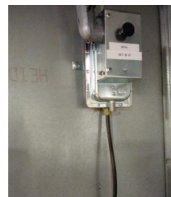
Static Pressure Sensor on Miriam AHU
