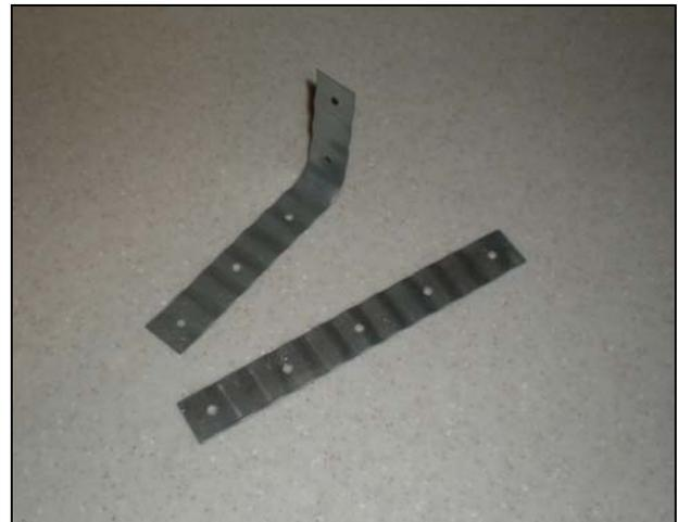
Figure 1 - Typical Corrugated Sheet-Metal Ties
