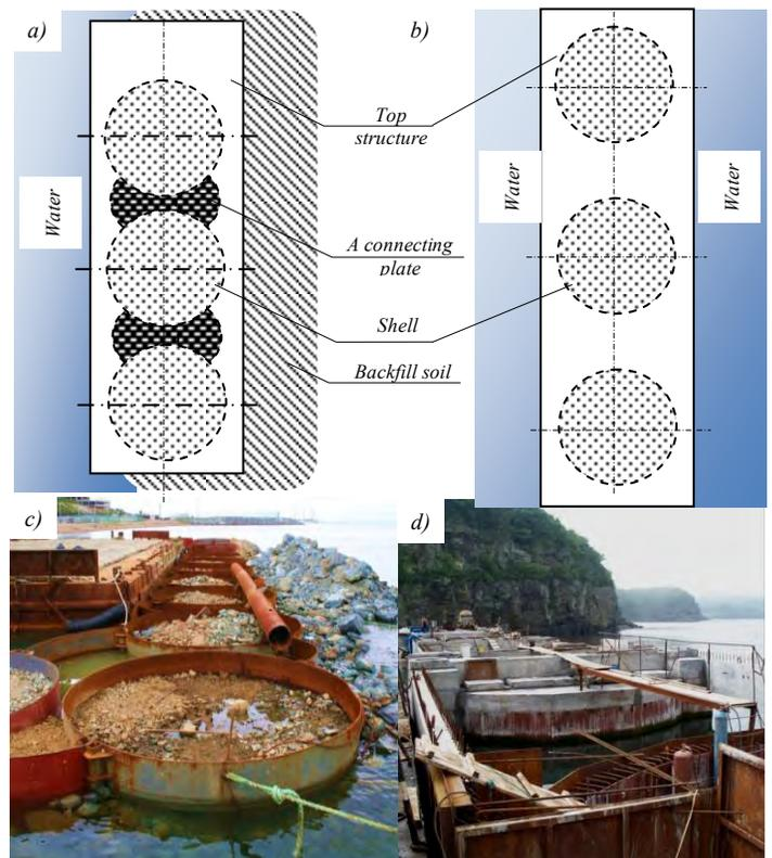
Fig. 2. Examples of large-diameter shell structures: a) a layout of a harbor wall (plan top view); b) a layout of a pier (plan top view); c) construction of a berth in the Fedorov Bay (Vladivostok, Russia) from steel shells with the infill; d) installation of the reinforced-concrete top
