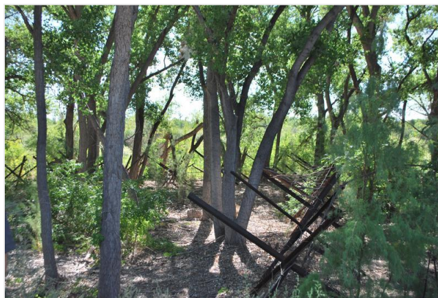
Jetty Jacks in the Bosquex
