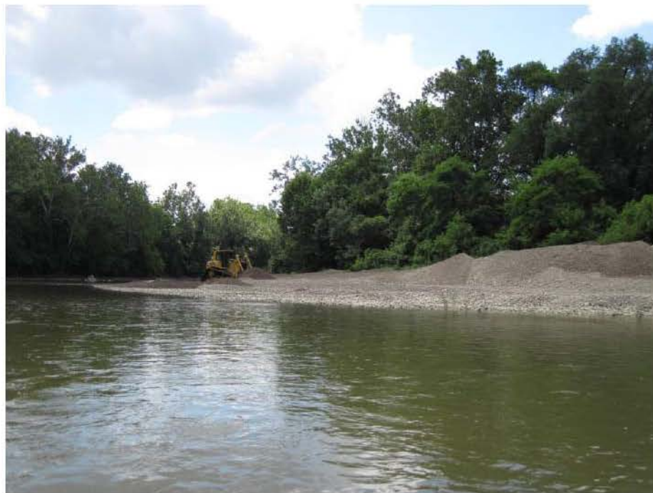
Unexpected construction on the river
