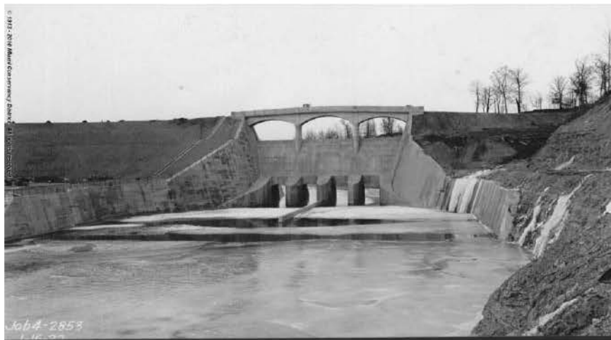
Fig. 6. Taylorsville Dam, taken 1/16/1922. View of downstream side from point on east bank, with a good view of spillway and bridge (Miami Conservancy District).
