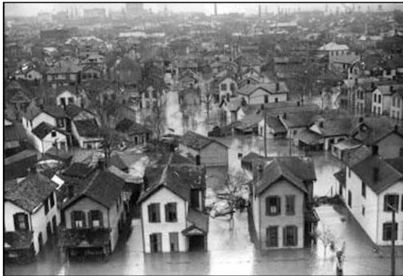
Fig. 4. “An aerial view from Miami Valley Hospital looking due north over Apple Street toward downtown Dayton begins to reveal some of the destruction to homes in the city’s southern sections due to the floodwaters’ powerful currents. Several homes have been moved from their foundations and so sit at odd angles with respect to their neighbors, and floating debris is clearly visible between houses” (Bell 2008).
