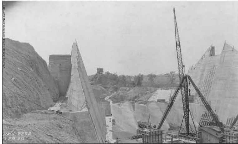
Fig. 5. Taylorsville Dam, taken 9/29/1920. View looking south, showing concrete in advanced stages (Miami Conservancy District).
