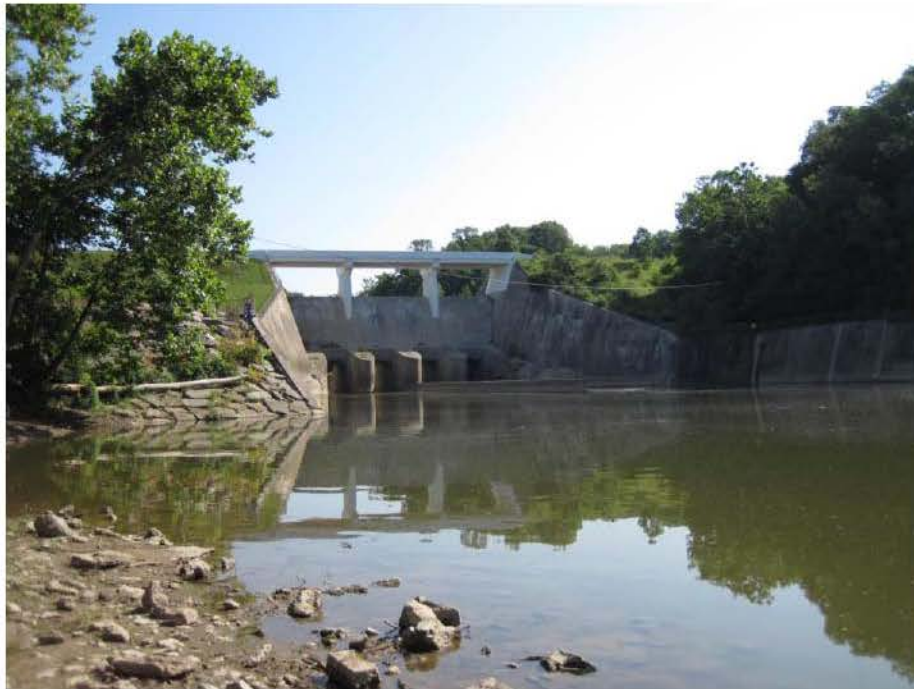
Downstream of Taylorsville Dam looking north
