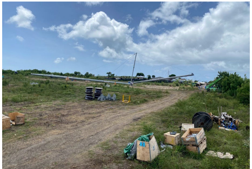
Figure 9: Construction Site of Hurricane-Resistant Wind Turbines. Source: [63]
